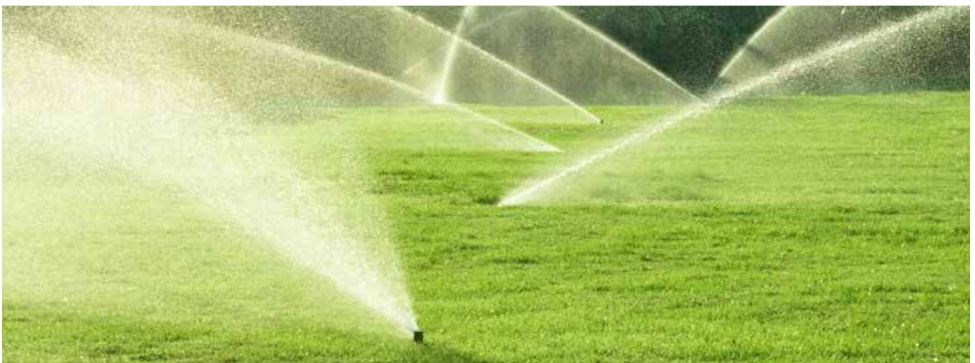
Automatic garden sprinkling system
