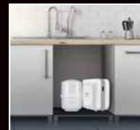
On The Floor Installation
